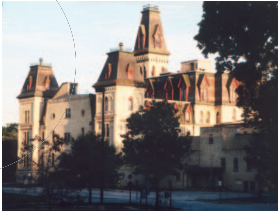
An evening sun illuminates the towers of the main domiciliary (1869), the signature building of the Soldiers Home, which once housed as many as 1,000 veterans. In addition, it held the dining hall and administrative offices. It was designed by Milwaukee architect William Townsend Mix and is an example of Second Empire Victorian work. At that time, Soldiers Home was located out in the country, and Milwaukee residents would catch a trolley or train to spend a day picnicking, visiting veterans, or seeing a performance in the theater there.
