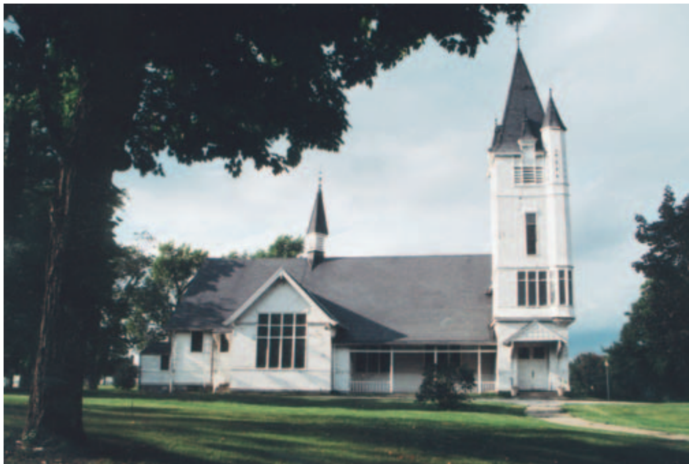
The multi-denominational chapel (1889) was built by soldiers who wanted a separate church structure and who contributed their own resources for its construction. Both Protestant and Catholic services were held there. It is in dire need of restoration.
