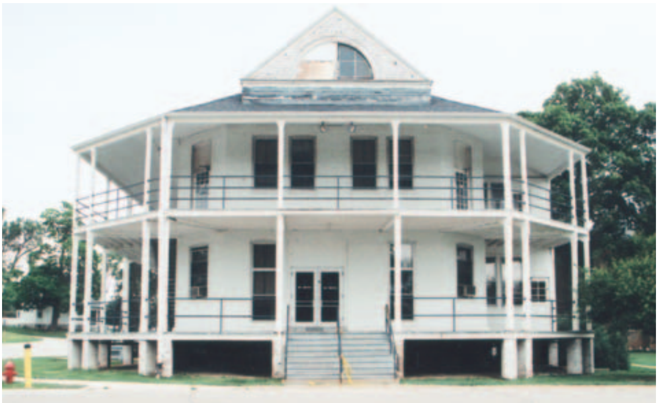
This is an end view of Building 6, a hospital and convalescent ward, built in 1879 and designed by Milwaukee architect Henry Koch, himself a Civil War veteran, who also designed Milwaukee's City Hall and Turner Hall. The third hospital on the grounds, it held elderly veterans for years, providing them with sun parlors filled with rocking chairs, easy chairs, writing desks, flower stands, canaries, goldfish, and early gramophones and radios. It held federal offices until July 2004, when it was vacated.
